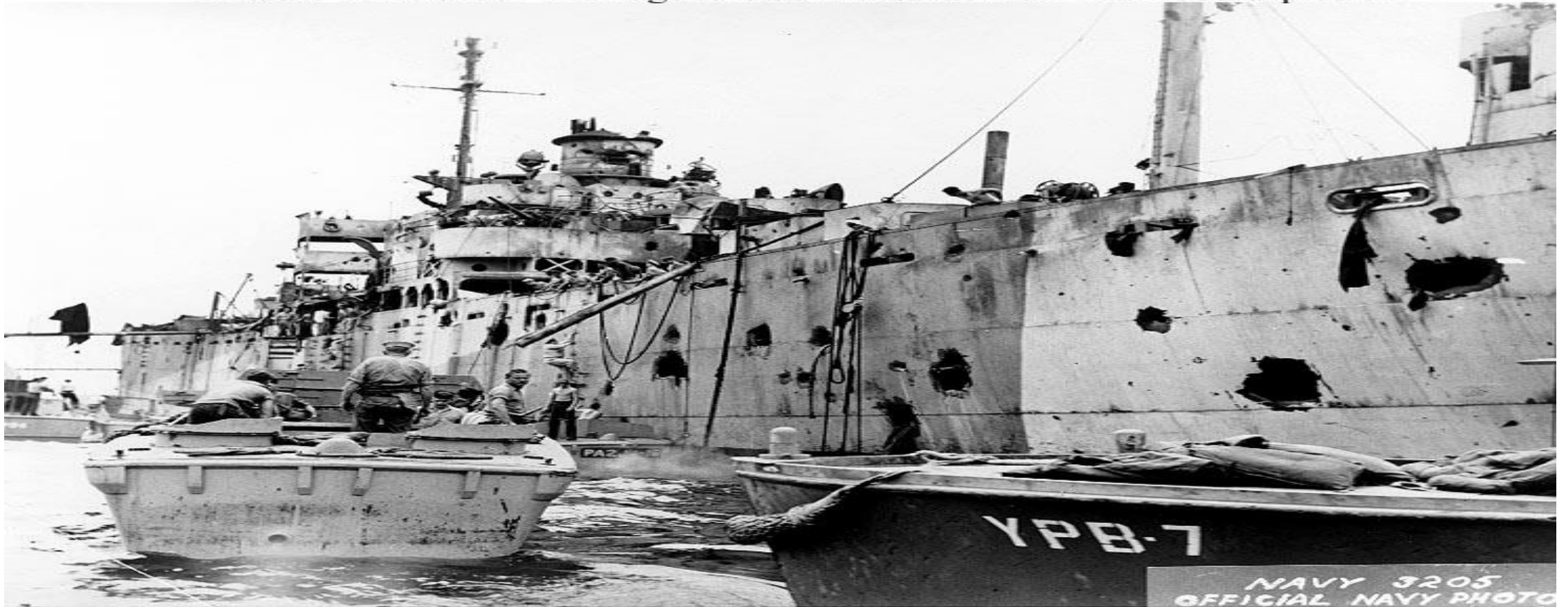
Photo # NH 96174 Damage to USS Mindanao from Mt. Hood explosion
